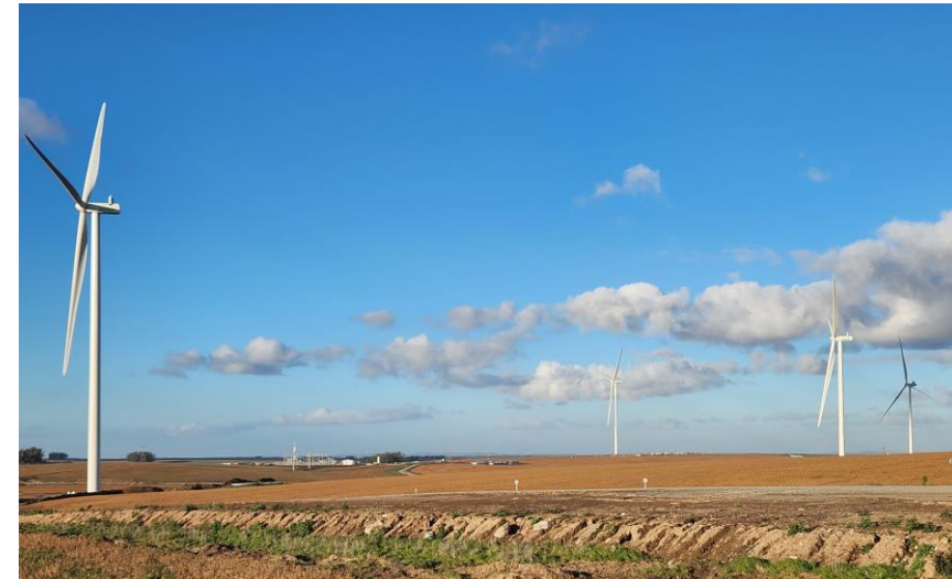
Photo: AMDA Consultants LLC
