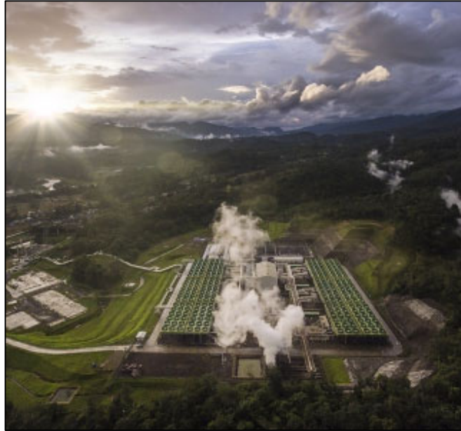
Figure 9.2: Sarulla Geothermal Plant, Indonesia
