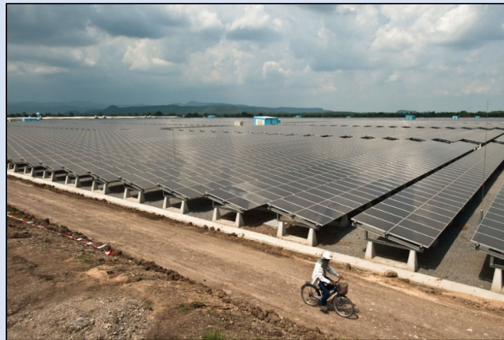
Figure 7.2: Central Thailand PV: Solar Power Project - Thailand's First Solar Power Facility
