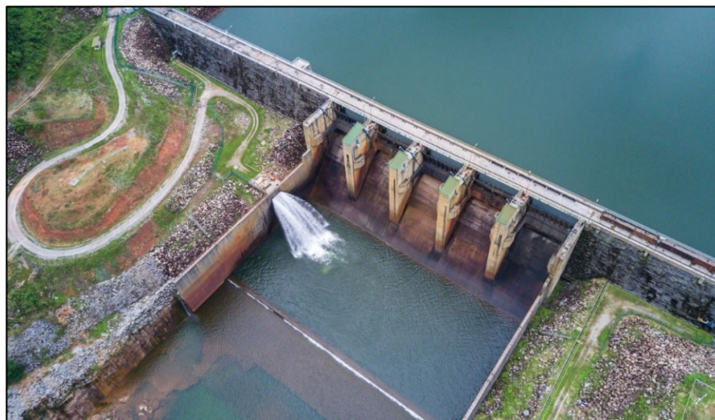
Figure 5.4: Dam at Nam Theun 2, Lao People's Democratic Republic, with downstream flow provision
