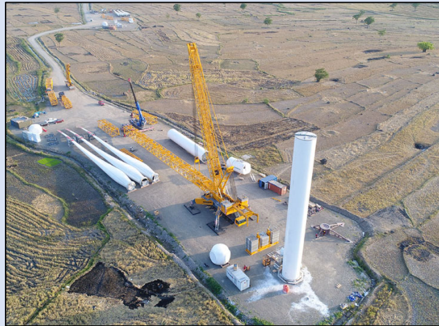
Figure 6.1: Construction of a wind turbine for the Tolo 1 Wind farm, Indonesia
