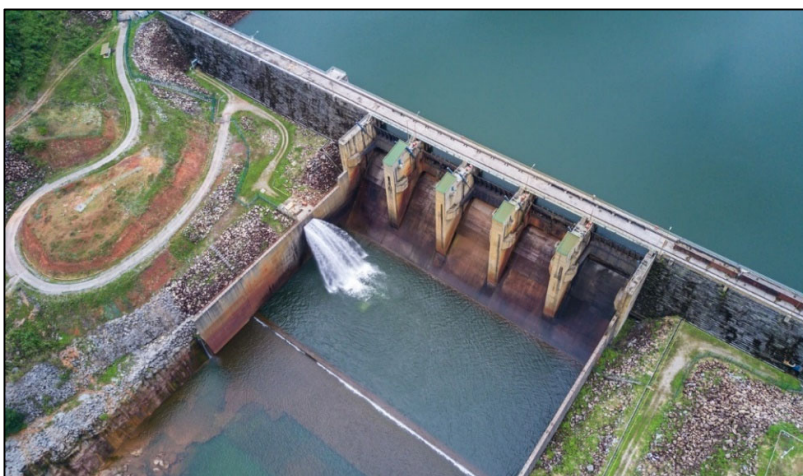
Figure 5.4: Dam at Nam Theun 2, Lao People's Democratic Republic, with downstream flow provision
